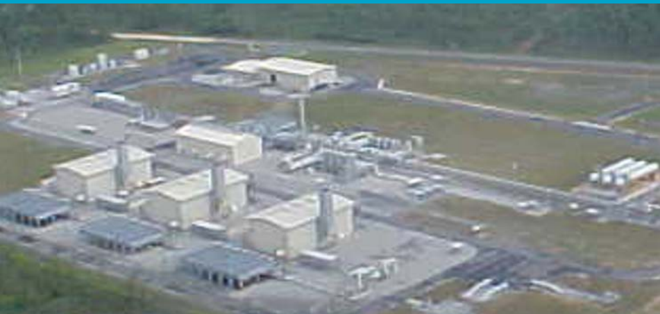
GULFSTREAM STATION 410 Alabama
